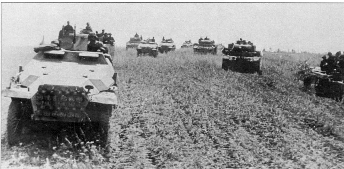
Here a formation of late production or reworked Pz.Kpfw. IV Ausf. Gs of 2.SS-Panzer-Division is accompanied by a Panzerbeobachtungswagen (Pz.Beob.Wg.) III artillery observation vehicle. These specialized tanks were very similar to the command tanks, being fitted with extra radio and observation equipment. Note that tactical markings and the national insignia have been painted on the wooden box added on at the rear.
