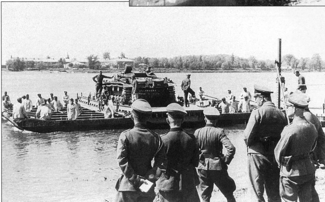
Here a StuG III Ausf. E of StuG.Abt.226 is being transferred over a river by bridge-building engineers. Four pontoons have been combined to carry a bridge section, thus creating a provisional ferry. Since the officers in the foreground seem quite unconcerned as they watch the activity, this was probably only an exercise.
